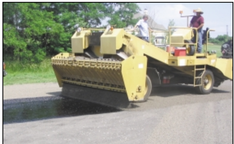
ASTM #9 LWA applied at 130 SY/CY over RS-1P Emulsion at 0.20 to 0.25 GAL/SY in a rural, residential cul-de-sac in Buchanan County, MO
