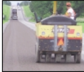
(Above) ASTM # 8 LWA applied at 115 SY/CY over CRS-2S at 0.40 GAL/SY in a county residential street • (Left) Pneumatic rubber-tire roller
