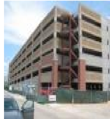
UofA Medical Parking Structure
